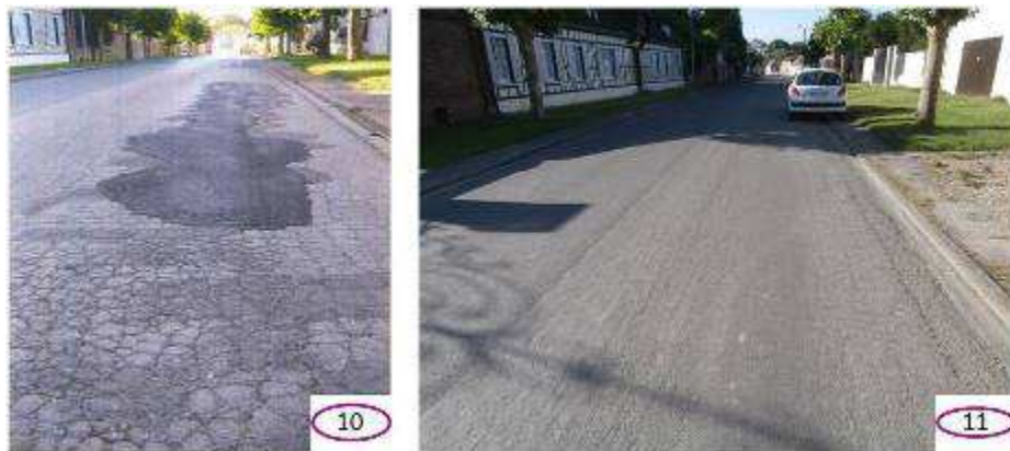
Figure 4: ARVILLERS: State of the pavement before the project and after 3 years of trafficking
