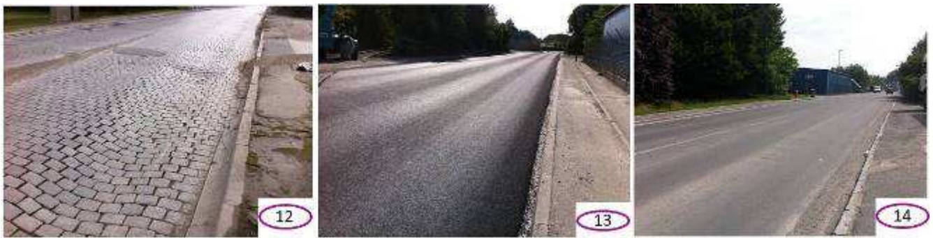
Figure 5: Port of LILLE: State of the pavement after 1 year of traffic
